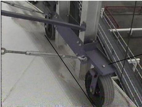
Make sure that the wheels are straight in line with each other Rather than turned to match the radius of the tank.
