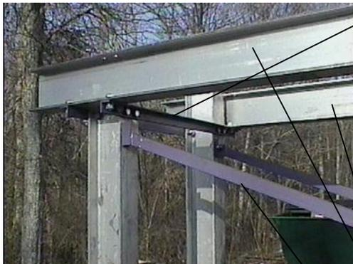
Bolt two Horizontal Angle Supports to each set of vertical beams. One on each side of the front beams, And one on each side of the rear beams.
