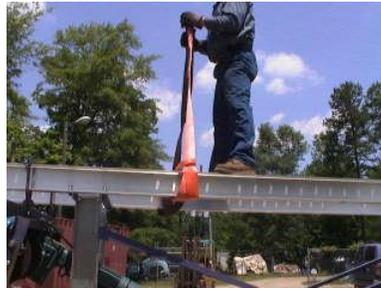
Use two straps to lift the fixture- one on each beam. Locate the straps about two foot back from the front vertical beams. Double wrap each strap so it won't slide along the beam during the lift. Pick the fixture off the ground, if it tips either way, readjust the straps so the unit picks up level. Caution- make sure the crane and straps are sized properly for the load. The fixture and the hoist weighs around 2000 lbs.
