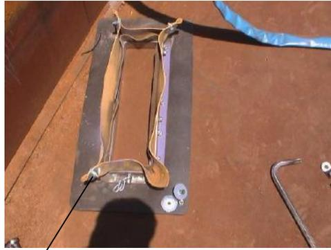
Clamp corners of the frame seal with 3/8" bolts
