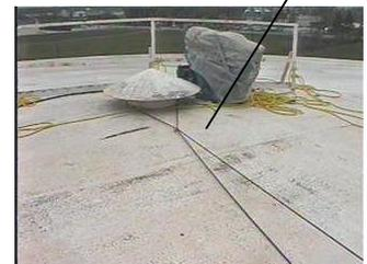
Caution- The center stand pipe must be structurally sound and capable of handling 1000 lb. pull at the base. The standpipe must be located in the center of the tank. If it isn't special cable connections must be made. Call RBW for help in set-up.
